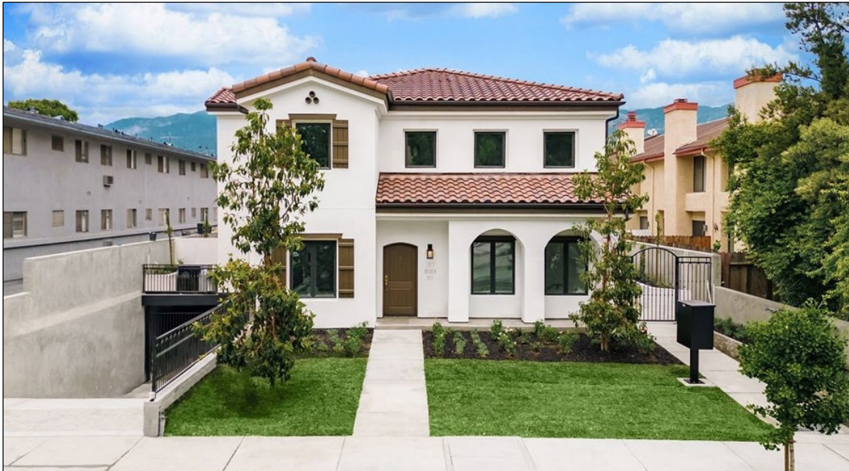
Figure 1 – Constructed multi-family units at 1027 Arcadia Ave.
